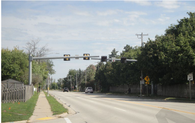
Pedestrian Hybrid Beacon (PHB) on Riverside Drive between West Briar Lane and St. Francis Drive.
