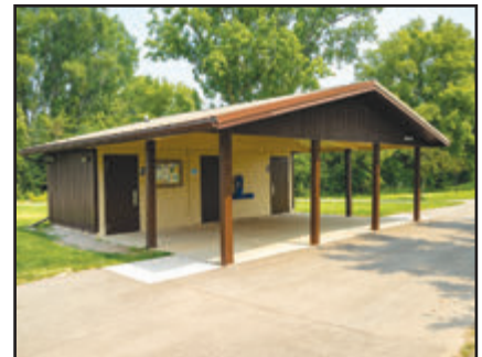
Kiwanis Open Air Shelter
