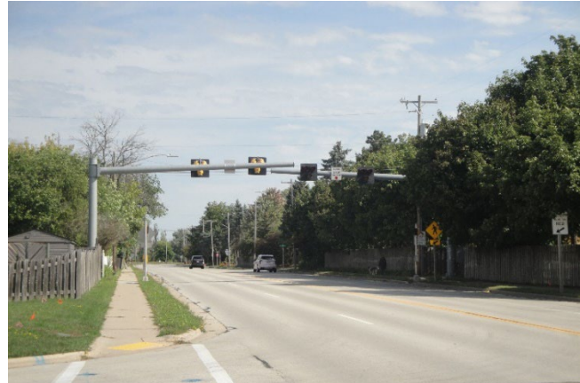
Pedestrian Hybrid Beacon (PHB) on Riverside Drive, north of West Briar Lane.
